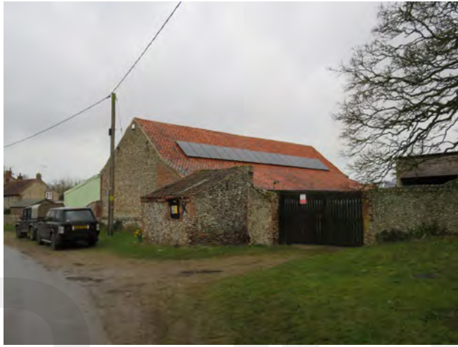
Solar panels on Church Farm barn
