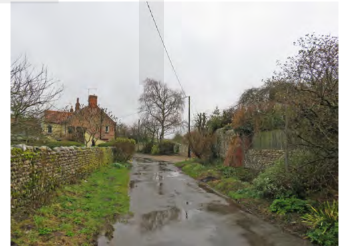
Electricity poles and cables deliver an essential service but detract from the appearance of the Conservation Area
