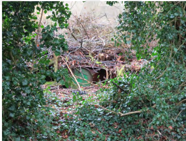
The storage of plants and unkempt grass detract from the streetscape whilst the trellis screening blocks the view towards Cley
