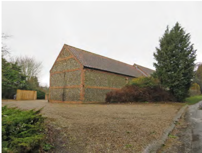
The access to the barn conversion on Hall Lane creates a gaping opening in the street boundary
