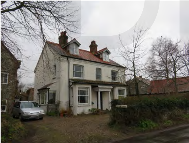
Climbing wall on the side of Glaven Lodge detracts from the appearance of the historic building
